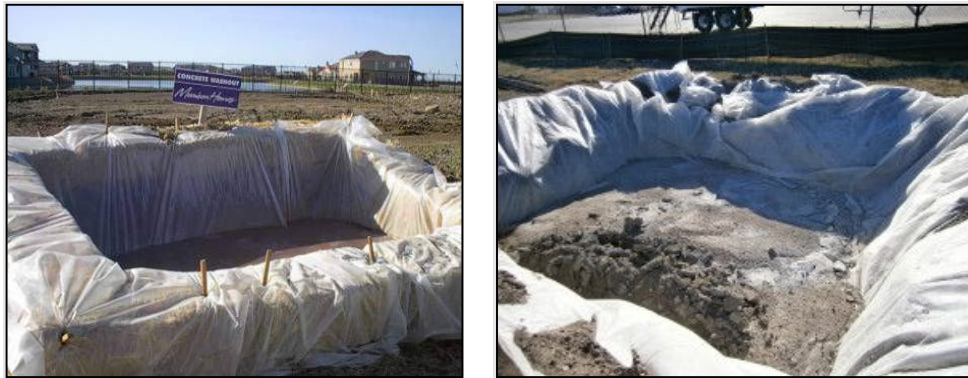
Plate 3-1 Typical concrete chute wash out areas
