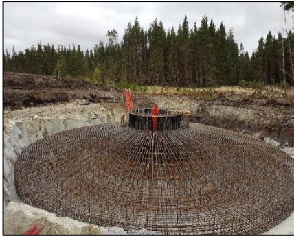
Plate 3.1 Turbine Base 'Anchor Cage'
