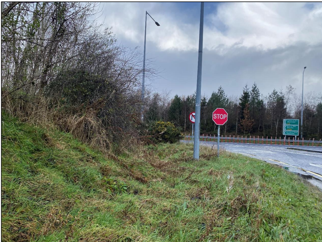
Plate 4-16. GS2 and WS! Recorded at proposed road widening area at the N5 and N17 junction
