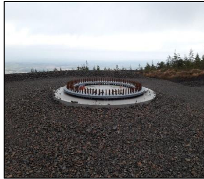
Plate 3.2 Finished Turbine Base
